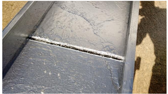
Figure 6: Drain With Overflow
